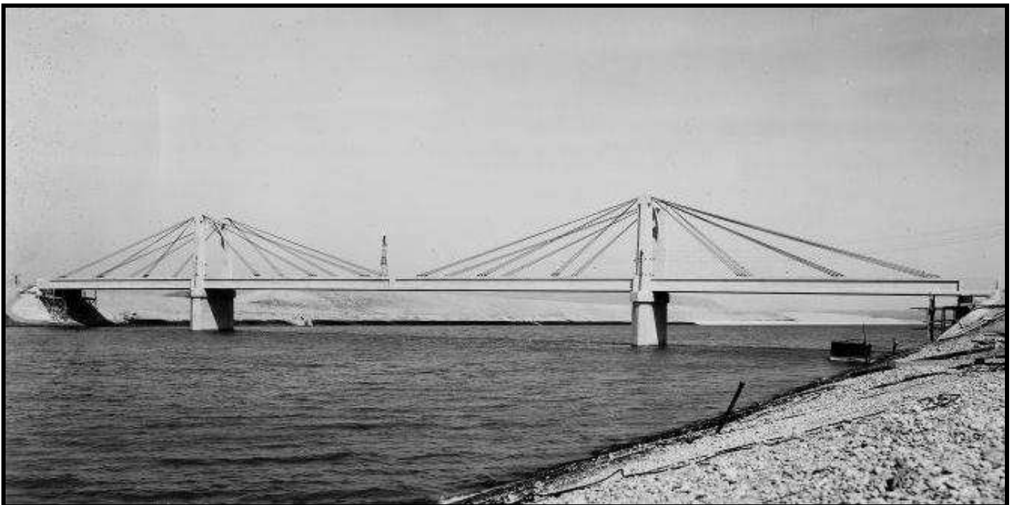
Cable Stayed Bridge
