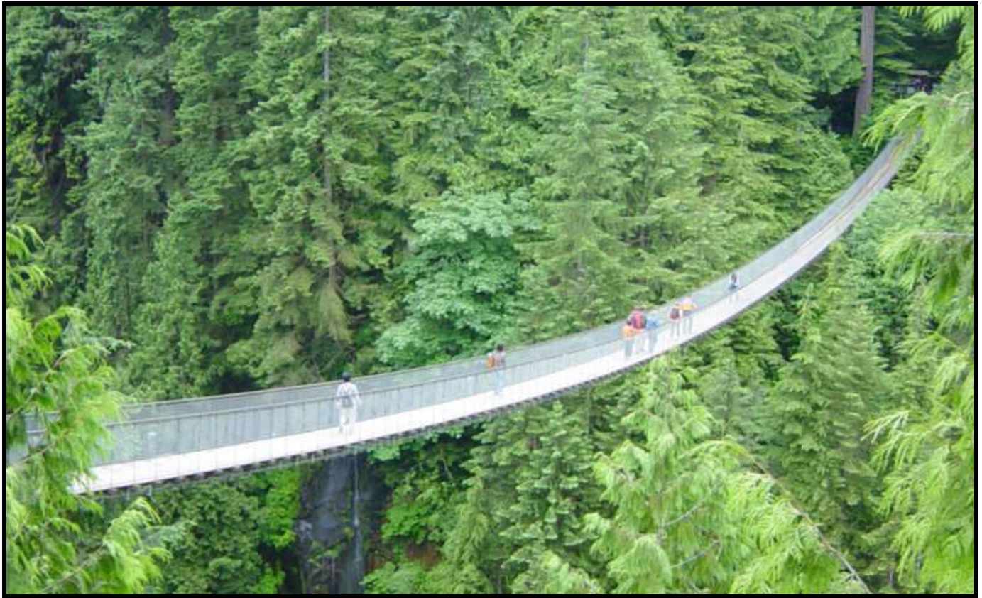
Simple Suspension Bridge
