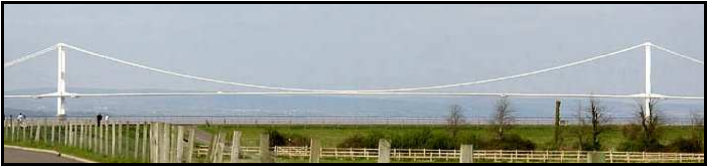
Hanging Deck Suspension Bridge
