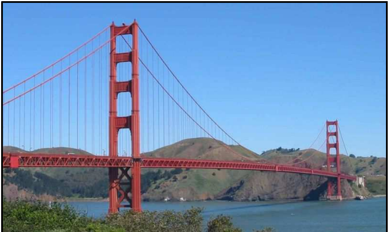
Hanging Deck Suspension Bridge
